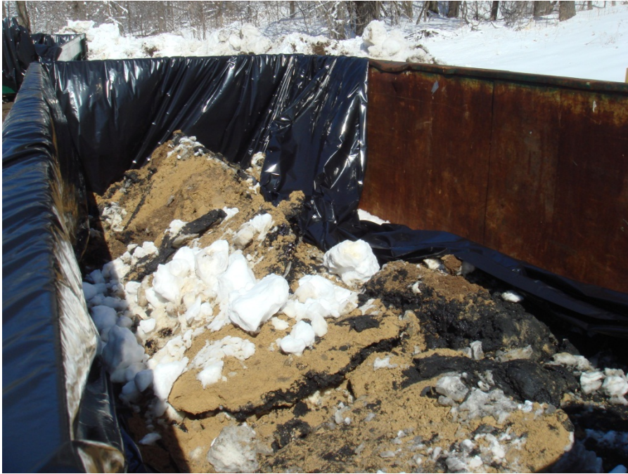
After water was decanted from the blower truck using a vacuum truck, the fuel oil waste
