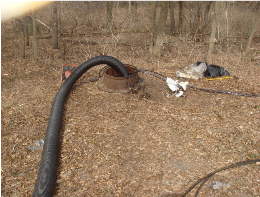
Typical sanitary sewer manhole between the METO and WWTP
