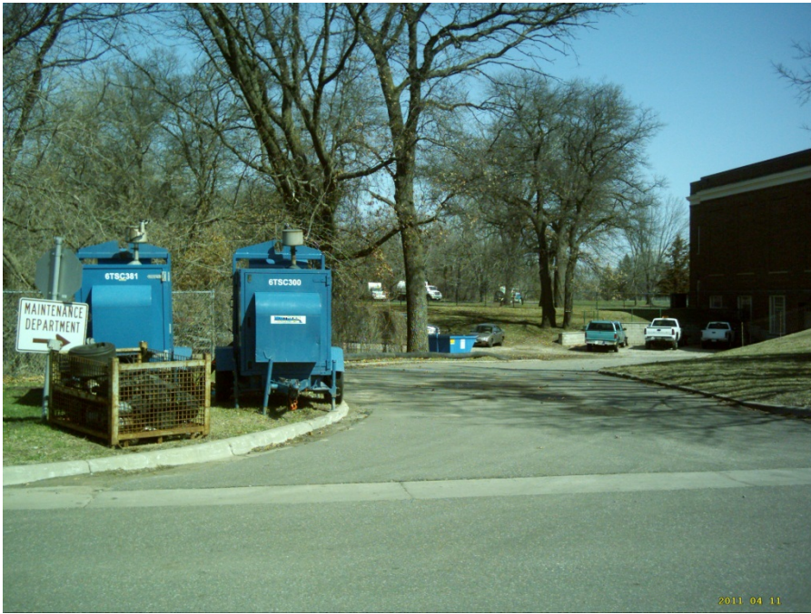
Sewage from the METO was pumped over the ground by the blue pumps shown to the left so that the half-mile of sewer could be cleaned
