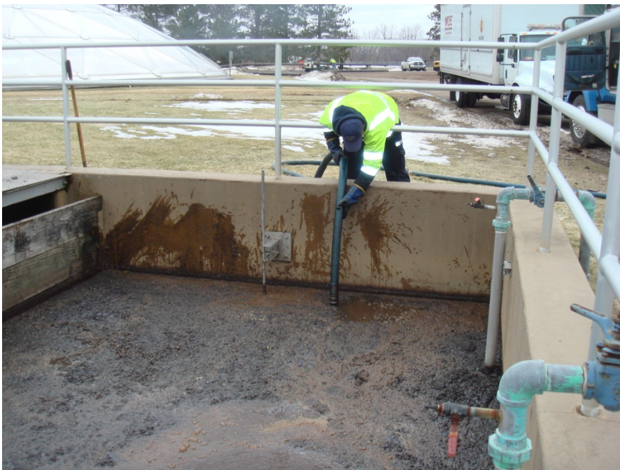
Cleaning RAS tank at WWTP
