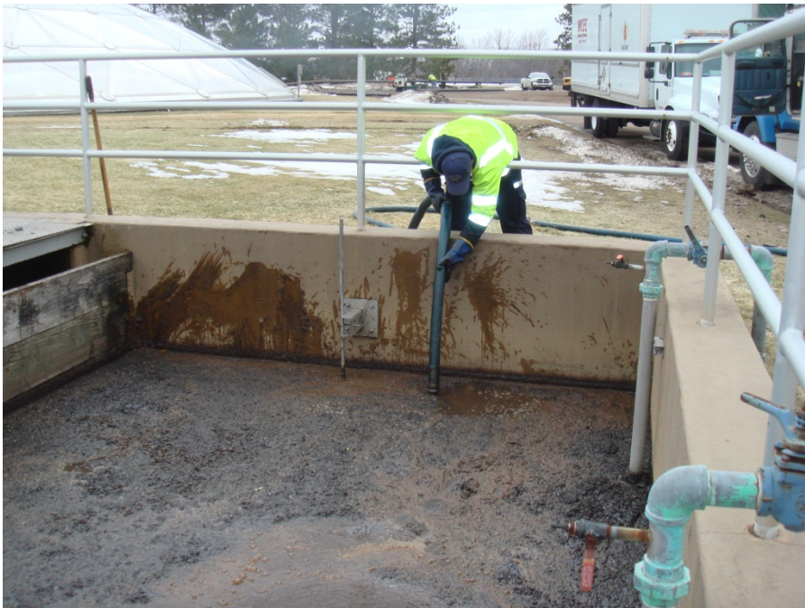
Cleaning RAS tank at WWTP
