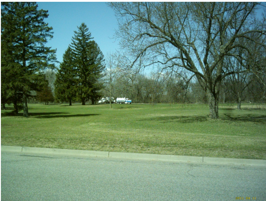
Vacuum trucks were used to recover fuel oil and jetting water from the sewer between the METO and the WWTP
