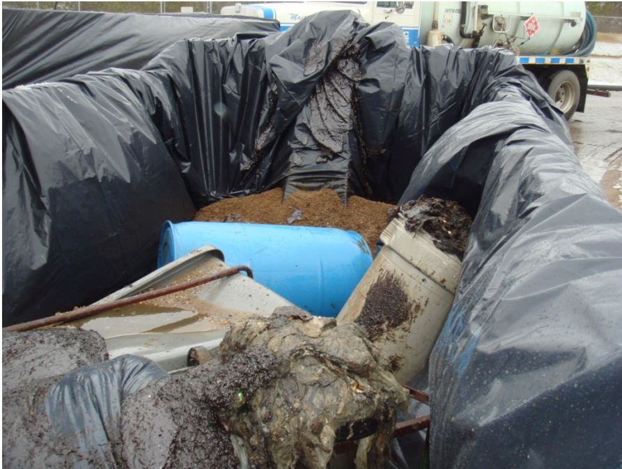
was mixed with sand, lime, and straw in roll-off boxes pending disposal
