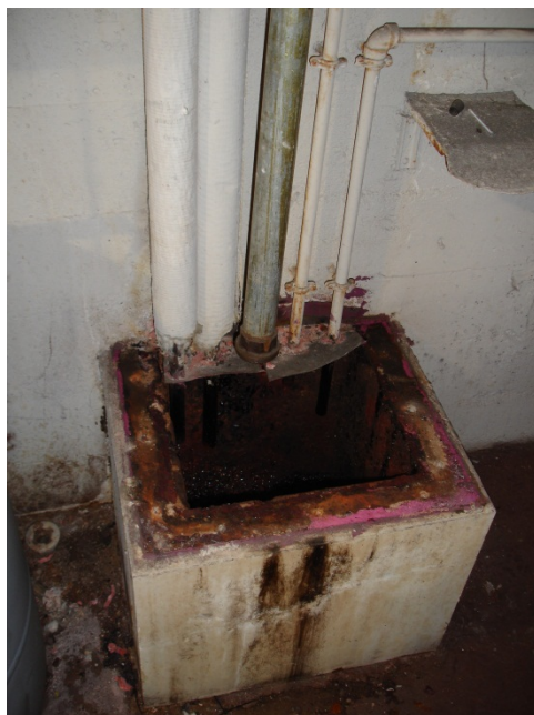
Piping at top of picture carries heating coil condensate water to floor drain at the power plant. The heating coils are necessary to make the fuel oil #6 flow.
