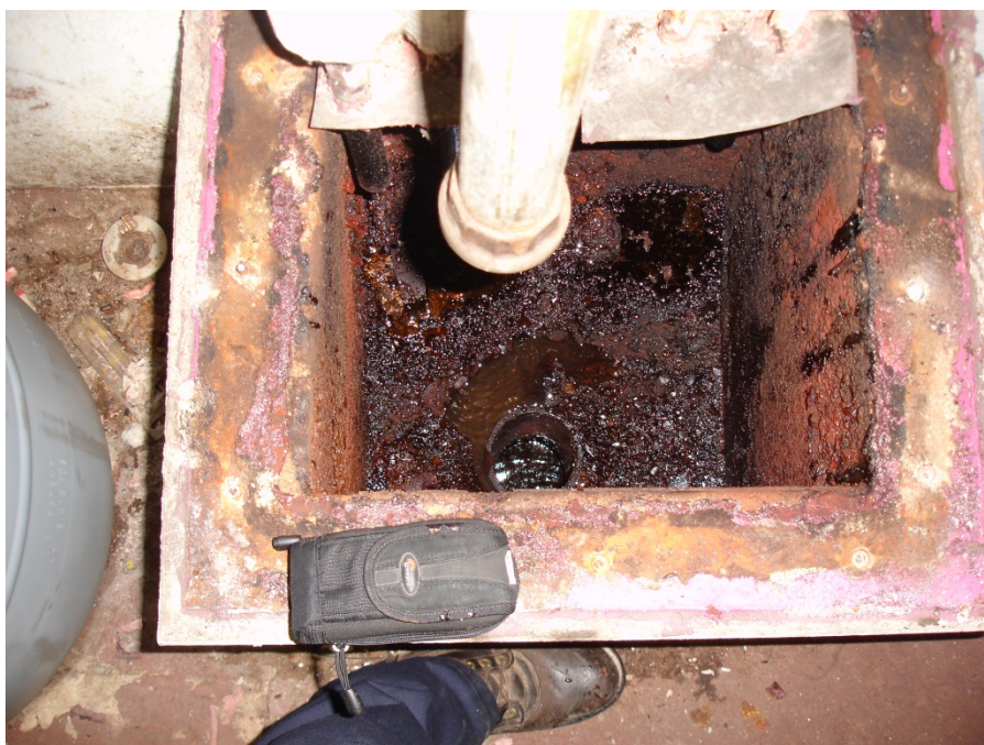
Fuel oil #6 entered corroded heating coils and flowed with condensate to floor drain that leads to sanitary sewer.
