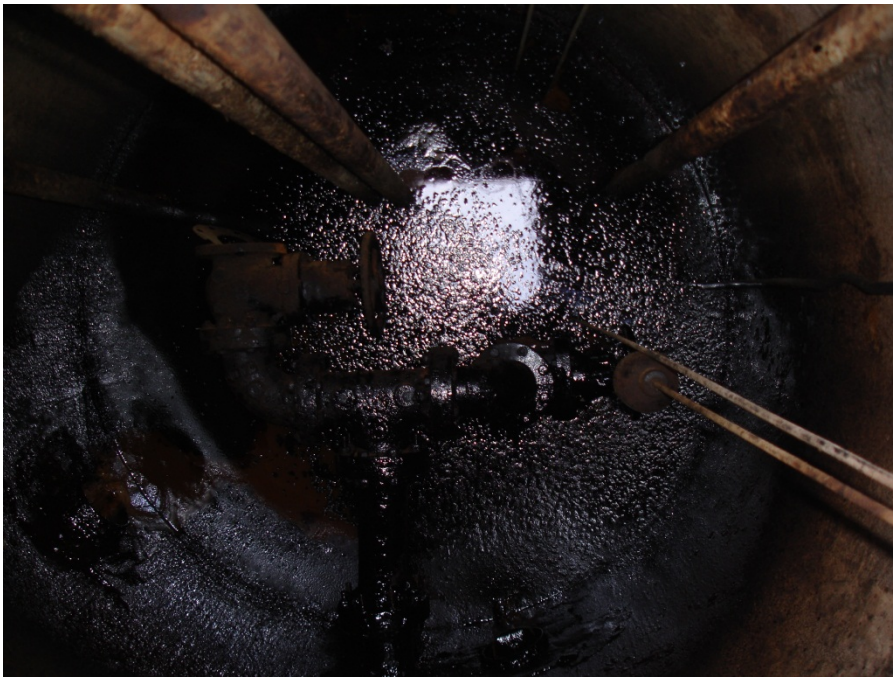
Oil in lift station located outside power plant. The lift station pushes sewage from the
