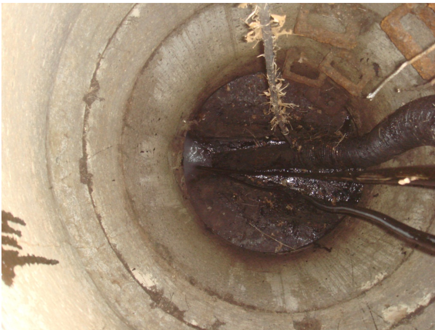
Vacuum hoses and jetter lines used to clean and recover fuel oil from the sanitary sewer
