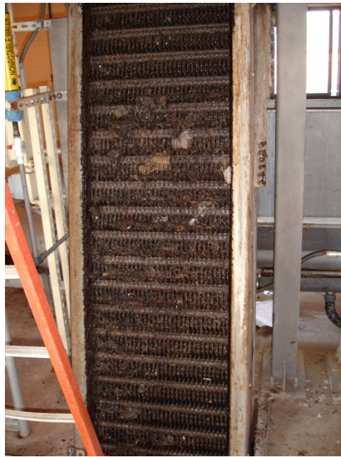
Fuel oil on waste conveyor at WWP pretreatment building
