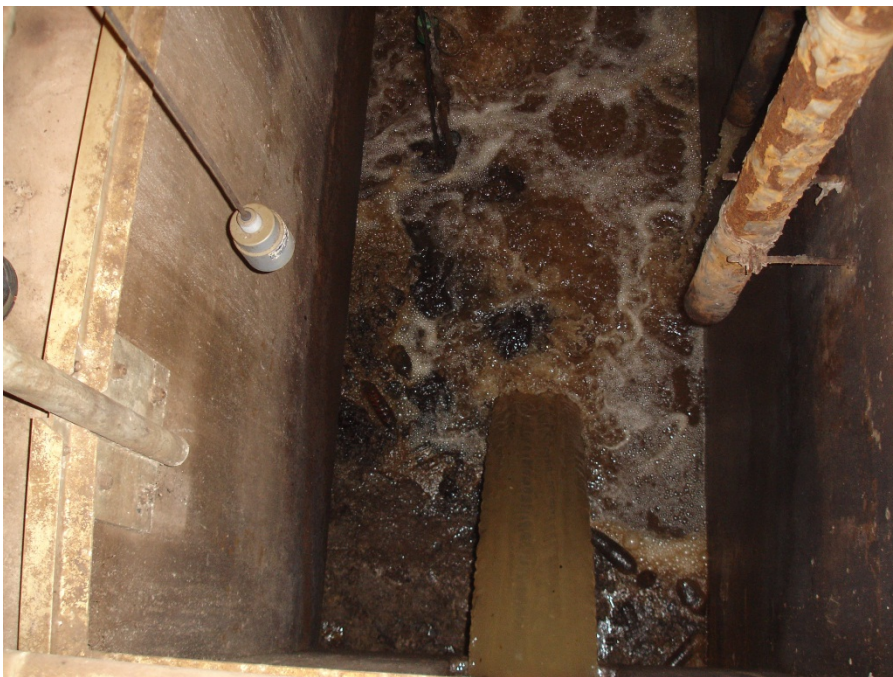
Deep pit or sump at WWTP pretreatment building contaminated with fuel oil
